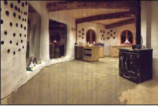
Adhering to the basic principles of a passive house the geodesic dome minimises heat loss and provides good air flow via the mechanical ventilation system. The passive solar gain, coupled with excellent thermal mass qualities of the thick COB walls, means it's easy to keep the house warm in the winter and cool in the summer. This passive house approach has resulted in better utilisation of energy and dramatically reduced heating requirements.
